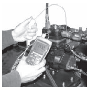
Testing the temperature at the discharge fitting.
