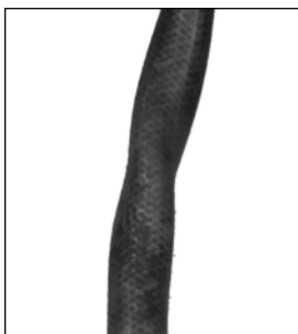
Partly collapsed inlet line shown.
