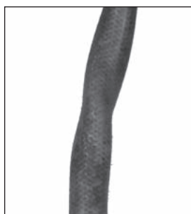
Partly collapsed inlet line shown.
