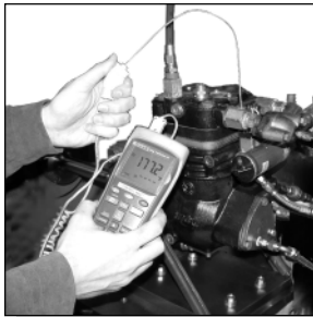
Testing the temperature at the discharge fitting.
